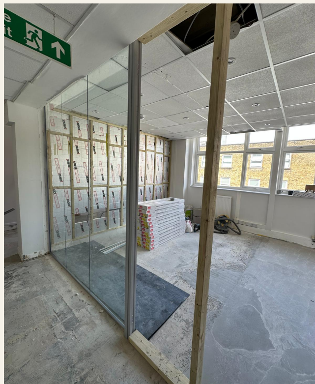
Partition works and floor preparation.
