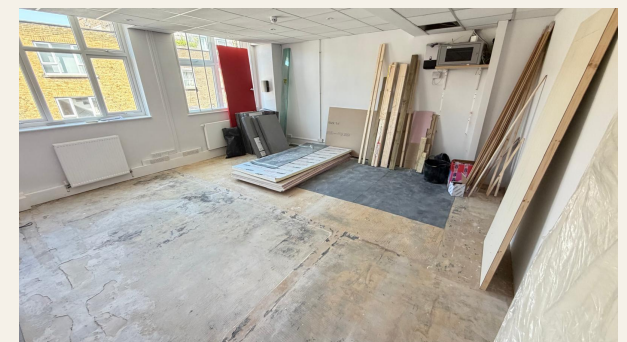
During / fit-out in progress
